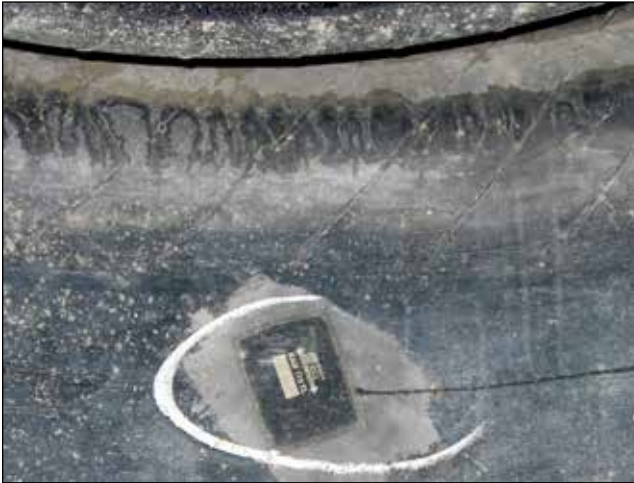
Improperly Aligned Repair (Note that the arrows on the patch do not point toward the beads.)
