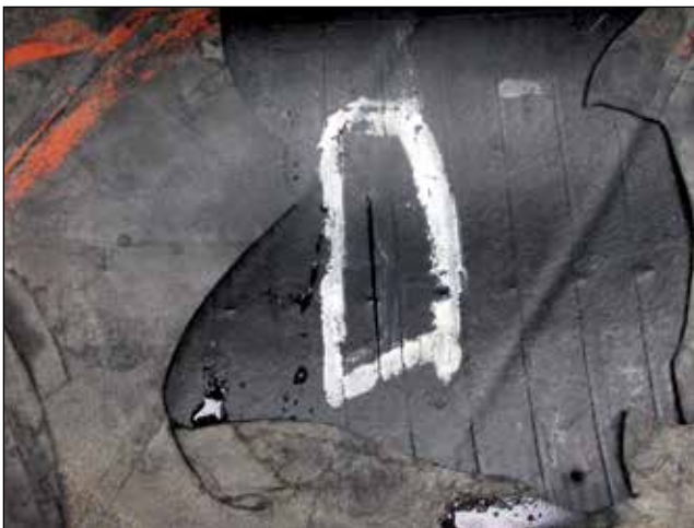
EFFECT: Radial Liner Split CAUSE: Due to Impact
