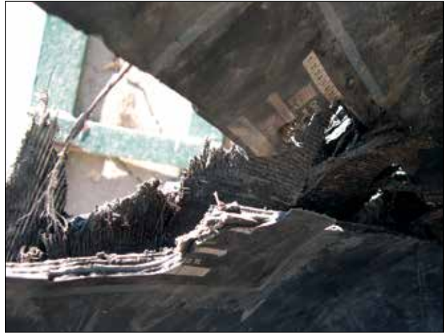
Rupture on Improperly Aligned Repair (Note that the arrows on the patch do not point toward the beads.)
