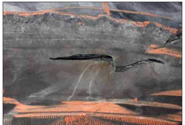
Sidewall Damage from Impact
