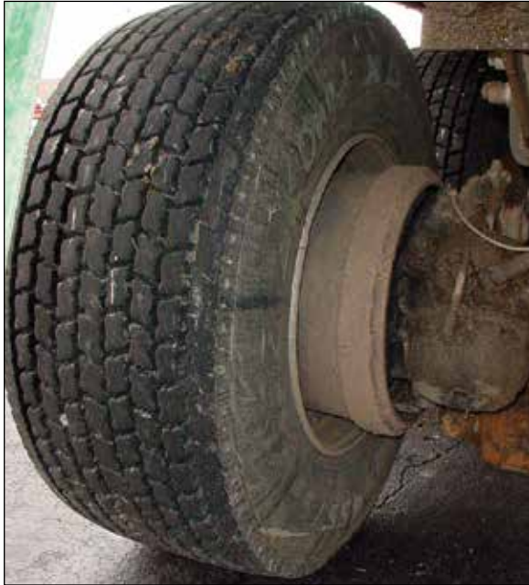
Exposed Brake Drum
